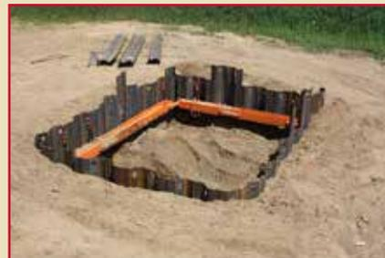
With all supports installed, connect the top level of the Pro-Brace to the bracing supports with Hanging Chains and pressurize system.
